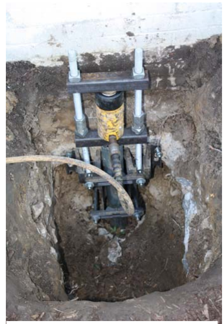
Hydraulic jack used to lift the structure
