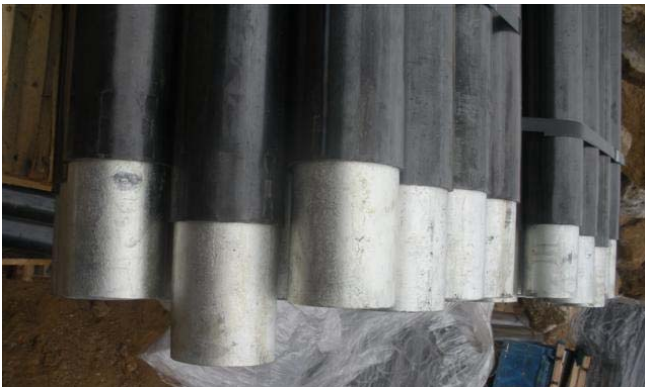
Couplings are crimped at one end of each pipe pile
