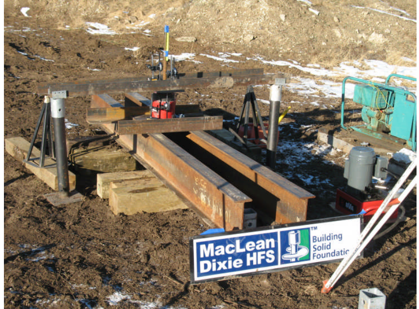
Pounds-force using a hydraulic cylinder to test pile in compression
